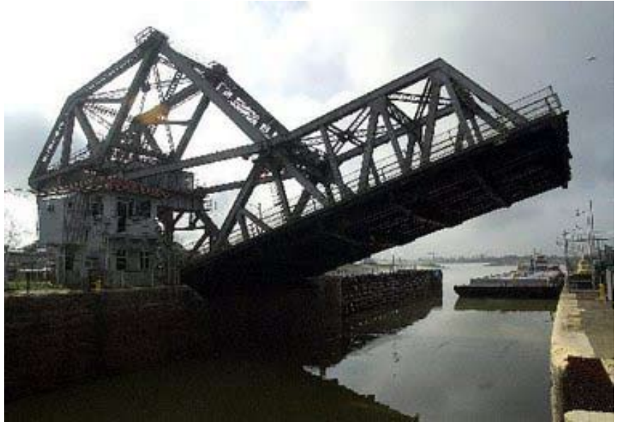
Figure 3: The drawbridge opening to allow a vessel through. Photo courtesy Chris Ganger, The Times-Picayune
