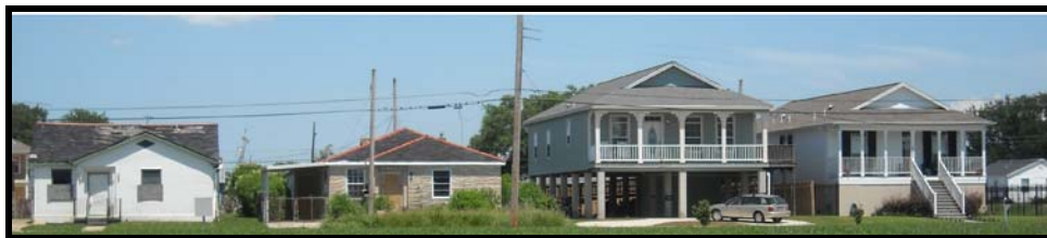
Figure 5 Unsafe and safer houses elevated post Katrina (see online version for colours)
