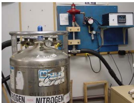
Liquid nitrogen tank
