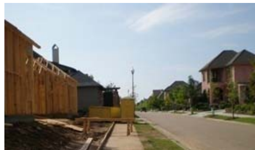
Image 3.25: Construction activity often blocks the sidewalks.
