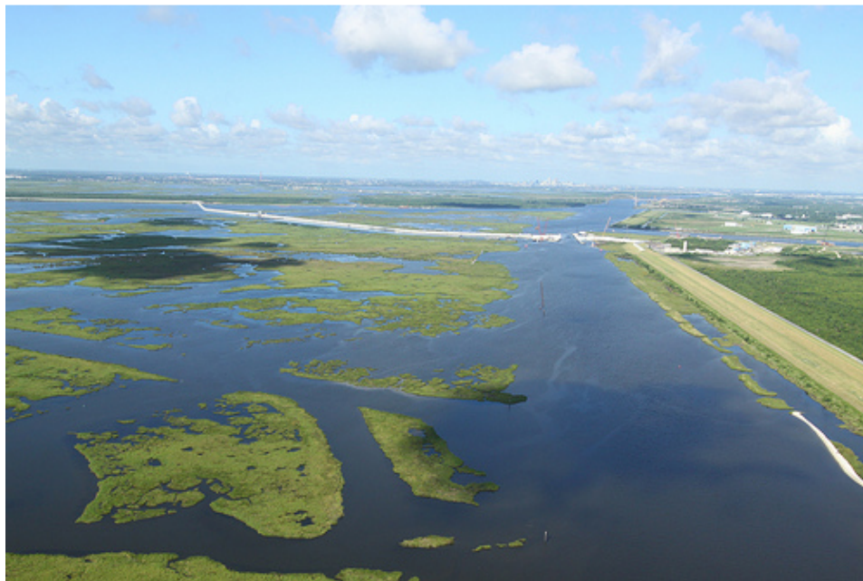
Figure 22. Image of completed surge barrier, with the MRGO to the far left and the IHNC on the right. The flood gates are visible in the photograph, with the gates in the open position allowing for boat traffic to continue in the waterway during normal conditions. In the event of a storm, these gates can be closed. (Image from Team New Orleans, Army Corps of Engineers http://www2.mvn.usace.army.mil )
