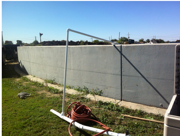
Figure 15. Pipe to remove excess of wastewater in the system.
