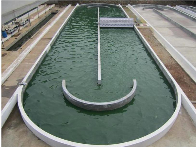
Figure 3. Raceways ponds. SOURCE: [www.aban.com](http://www.aban.com)
