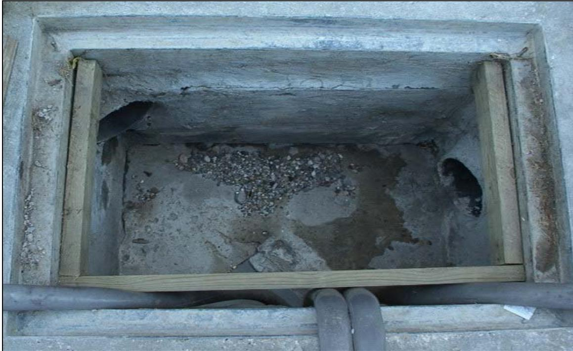
Figure 6: Drainpipes in Manhole from which the Highway Runoff is Collected.
