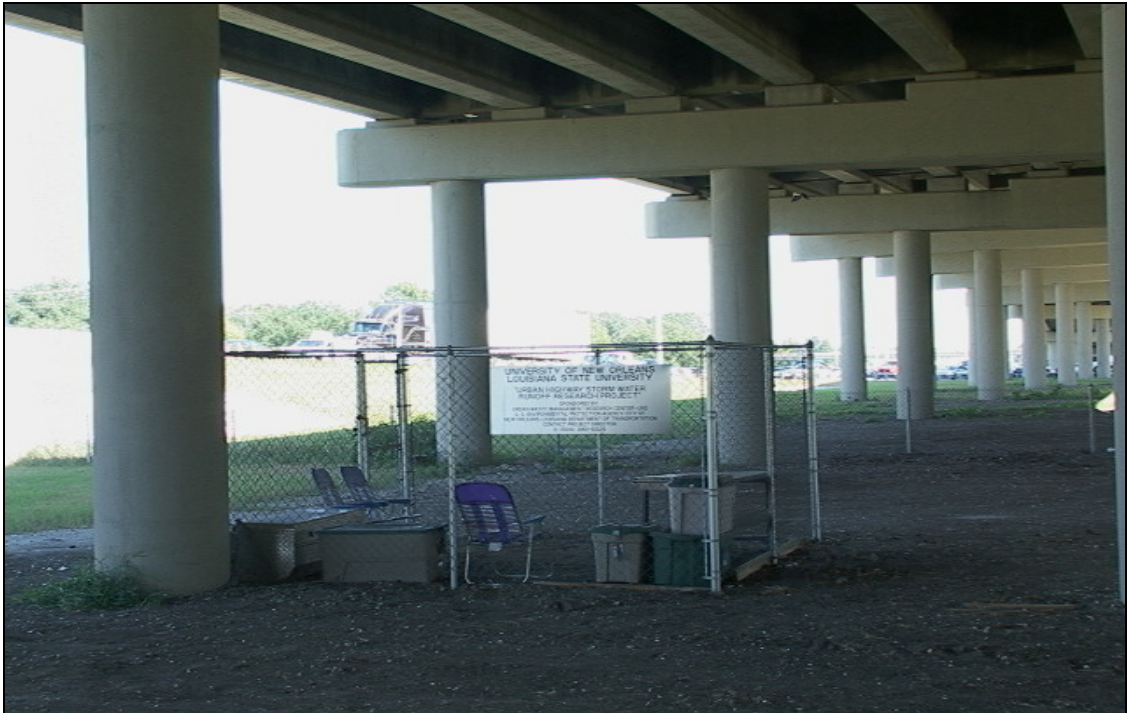
Figure 4: The Experimental Site Beneath the East-Bound Lane of the Interstate-610.
