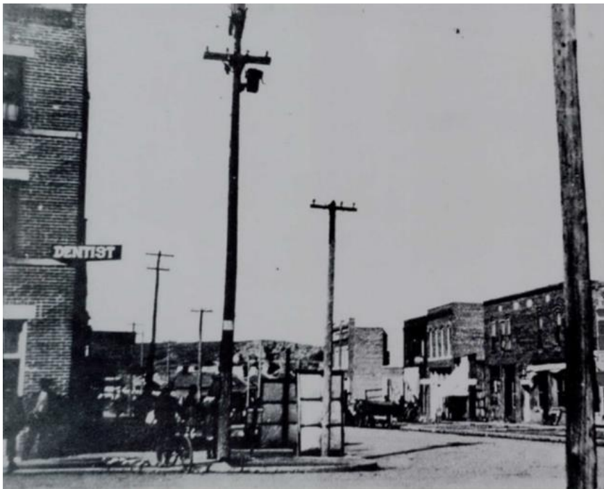
Figure 3: North facing views from Greenwood 1917, Tulsa Historical Society
