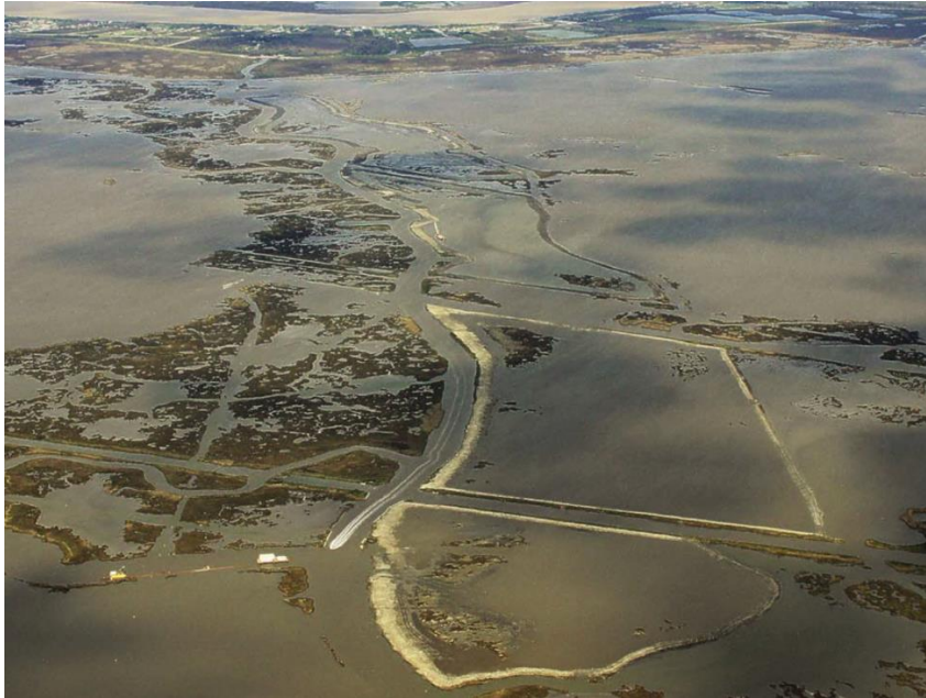
Figure 1.6: Marsh Creation site aerial photo (Credit: CPRA)
